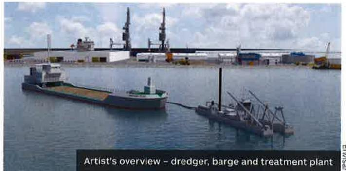
"The remaining volume, along with approximately 10,000 m<sup>3</sup> that was dredged from the Kanalen Grilstad port, has been stored in submarine cells that have been completely closed off. The project was delivered successfully in June 2016."
