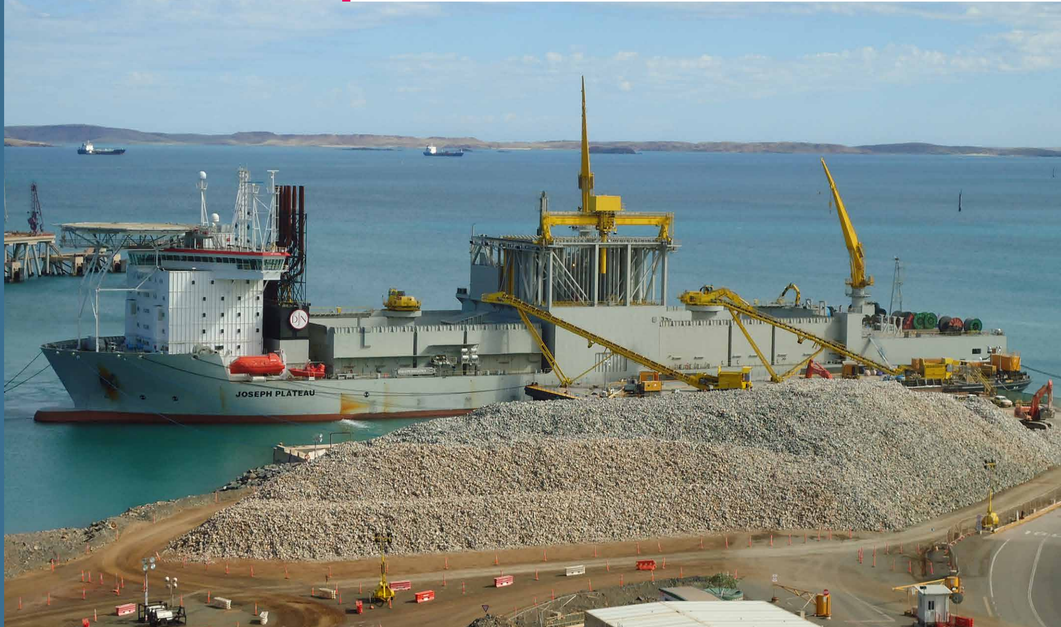
DP2 Fall Pipe Rock Installation Vessel
