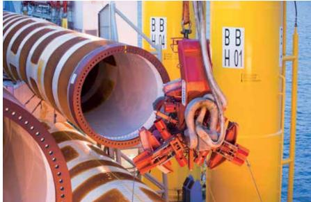
The entire WTG structure consists of a large-diameter, thick walled, steel monopile driven into the seabed by using the hammering technique, a transition piece which is bolted to the monopile, while the WTG consists of a tower, nacelle with generator and 3 blades.
